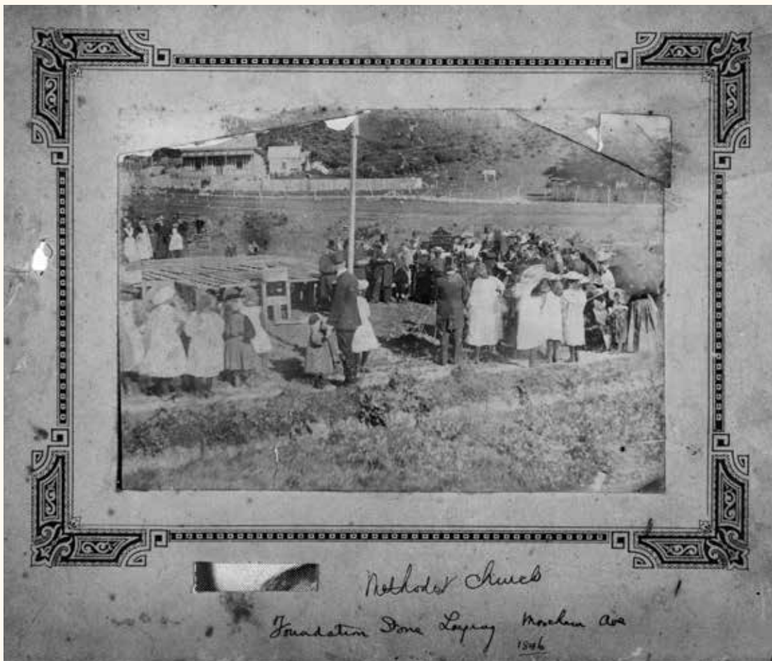
The laying of the foundation of the Wesleyan Methodist Church in Moxham Avenue, Hataitai (or Kilbirnie), Wellington, in 1896. The church was part of the Wellington circuit, where Josiah Ward was the main minister, and he is probably the speaker while Mrs Ward is seated at the harmonium. The church seated 100 people and was built beside the state school for the sum of £39.15 using donated materials. ALEXANDER TURNBULL LIBRARY. REF: 1/2-075654-F
